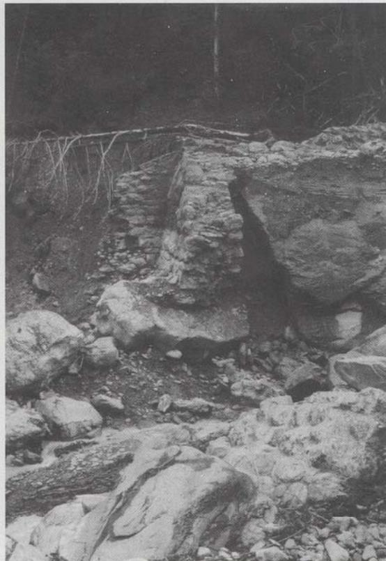
Fig. 6. Check dam destroyed in the Barranco de Arás gorge. The large boulder on which the dam was founded was undermined and displaced. Flooding waters partly eroded the ground behind the abutment. Some infill deposits are still visible upstream the dam (right).
