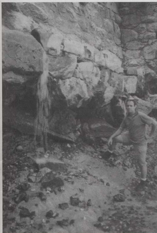
Fig. 5. Check dam undermining upstream check dam CD-2. Waterfall eroded ca. 2.5 m of till.
