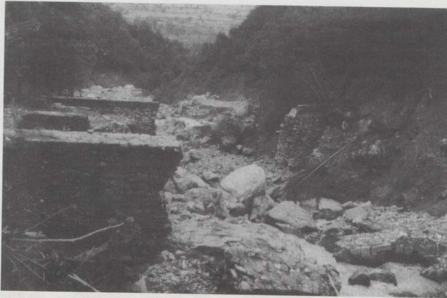
Fig. 4. Check dams destroyed at the Barranco de Arás gorge, downstream of check dam CD-1. Remnants of the former surface of the dam infill are observable on the right hand side of the barranco (center of the photograph).
