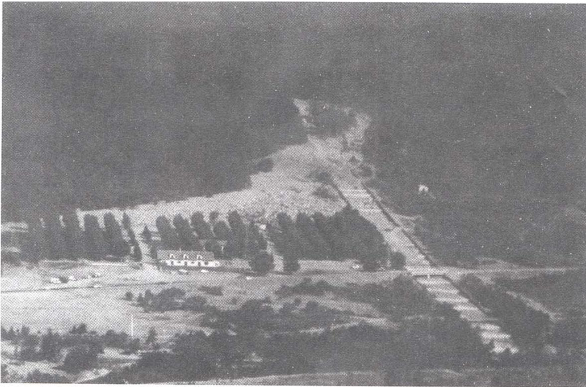
Fig. 2. The Barranco de Arás fan and Las Nieves campsite two weeks after the 7 August 1996 flood. On the right, there is the stair-shaped artificial channel. Close to the fan apex, the flow abandoned the artificial channel, hit the rock spur, crossed the artificial channel and followed its former natural channel behind the campsite. Water flooded the fan between both channels.
