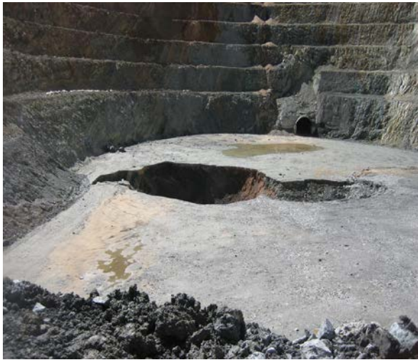
Figure 5. Subsidence in the bottom of Tinyag mine
