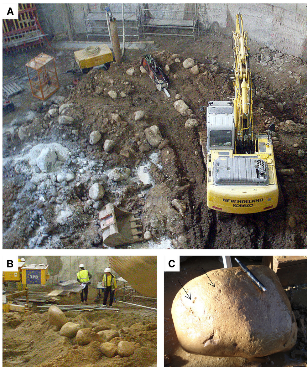
Fig. 4. Excavation of the shaft-station of Foc-Cisell. (A) General view of the removed layer of boulders in the shaft; (B) detail of some boulders showing its characteristic well rounded shapes; (C) detail of a single boulder showing small borings (arrows) made by lithofagous fauna.
